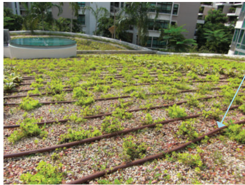
Fig 1: A typical drip-type irrigation system laid on the surface of the substrate of a green roof system.
