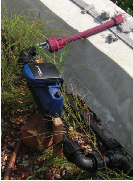
Fig 10: A typical controller of a drip irrigation system
